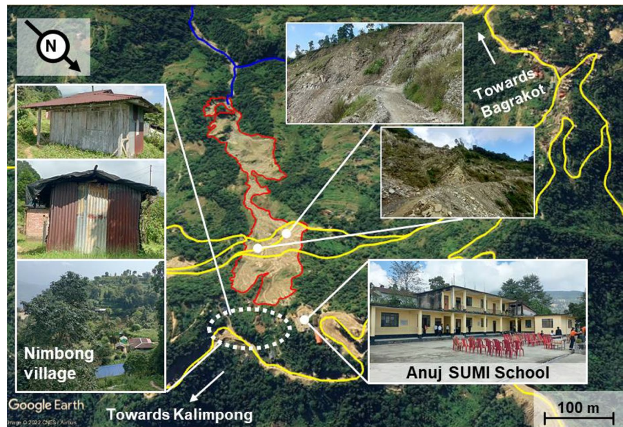
Fig. 1 Aerial view (Google Earth image) of the Zero landslide with associated risk elements
