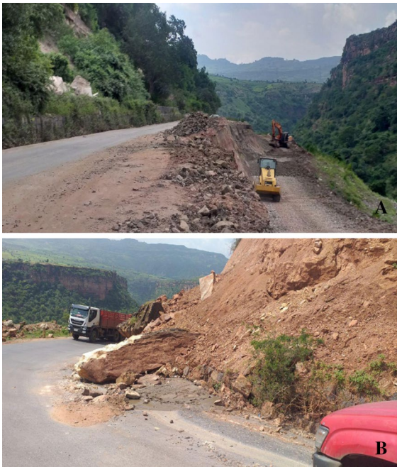
Fig. 6 Photographs showing maintenance of the A roadsides slides, and B rock slides
