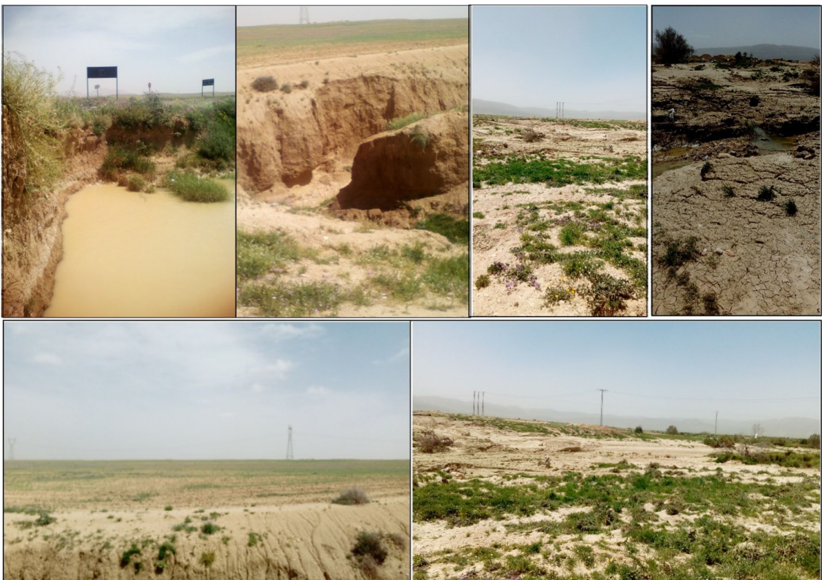
Fig. 1 Photos of some disasters caused by the effect of water erosion
