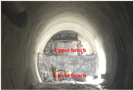
Fig. 8 Excavating by benching method in shanyang tunnel
