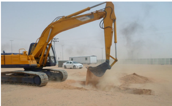
Fig. 4 Poklain during excavation of trial pit at proposed location in Sultana
