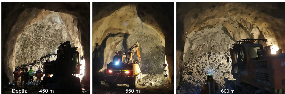
Fig. 13 Excavation faces along the adit at various depths below ground surface
