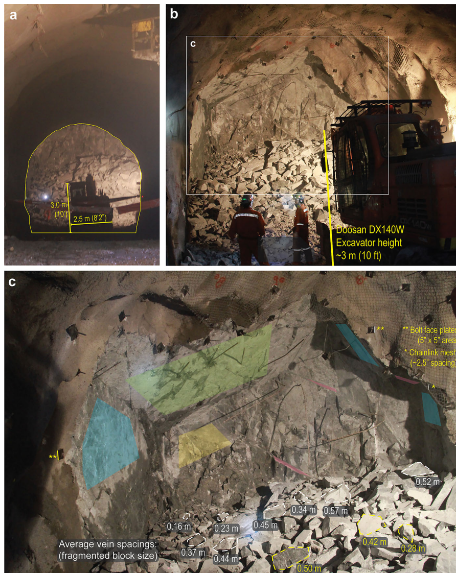
Fig. 14 Site observations from the 600 m deep excavation face of the adit at El Teniente. a Approximate excavation profile of adit approximately 5 m behind the face; b view of excavation face including immediate roof; b detailed view of excavation
