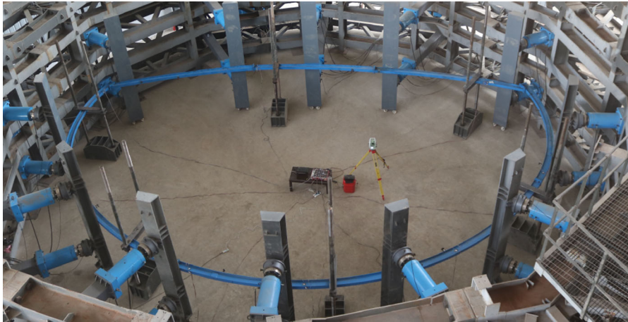
Fig. 6 Placement result of arch
