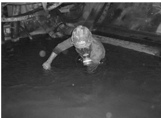
Fig. 4 Excessive water flow and the harsh environment at the Zagros tunnel. (Courtesy of Mirmehrabi et al. 2010)
