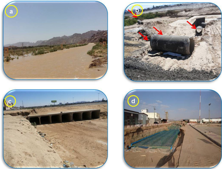
Fig. 13 a Some examples of flash flood problems in Wadi Najran 2016, b damages to the urban infrastructure, c and d underground rainwater drainage systems design in the area that are subjected to floods
