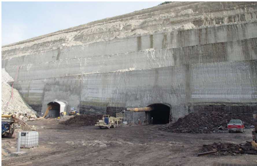
Fig. 6 View of the main mine entries
