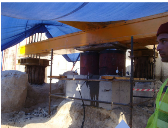
Fig. 2 Static load test in the future Etisalat center
