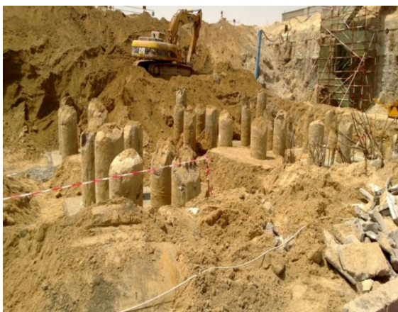
Fig. 1 Piles underneath the future Etisalat center in Abu Dhabi
