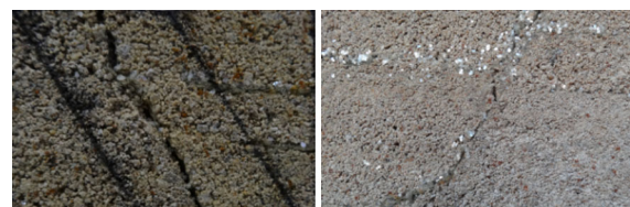
Fig. 14 The throughgoing fracture on the surface of the fault zone
