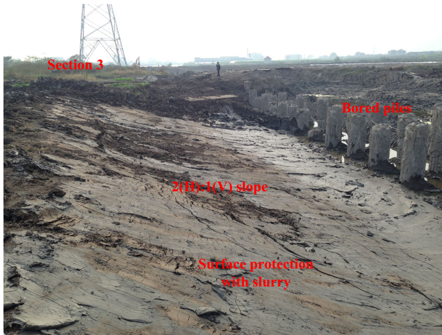
Fig. 5 View of placement of the bored piles and excavation phase 1
