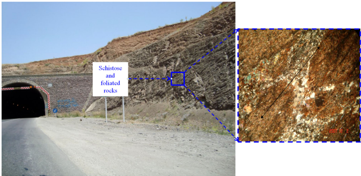
Fig. 6 Rock mass schistosity in the tunnel area. Courtesy of Ebadi (2011) and Ghasemi et al. (2007)
