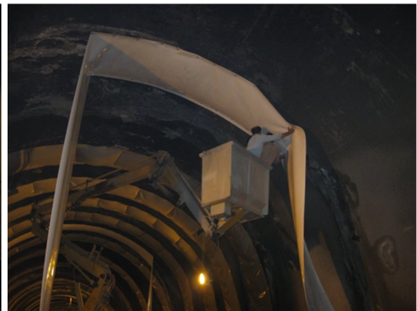
Fig. 5 The permanent lining of the tunnel. Adopted from T.S. Courtesy of Aria (2016)
