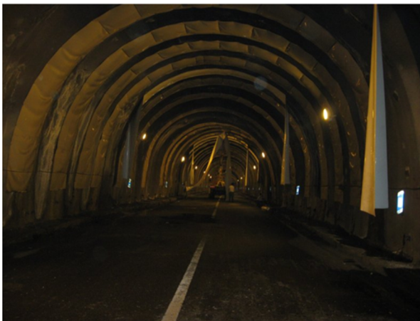
Fig. 5 The permanent lining of the tunnel. Adopted from T.S. Courtesy of Aria (2016)
