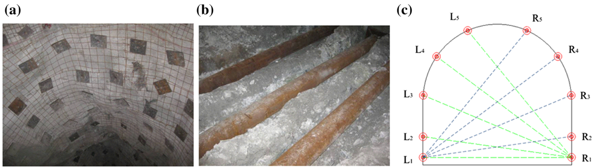
Fig. 6 Construction procedures: a installations of fully grouted bolts and nets; b installations of steel pipe beams on the floor; c locations of monitoring points
