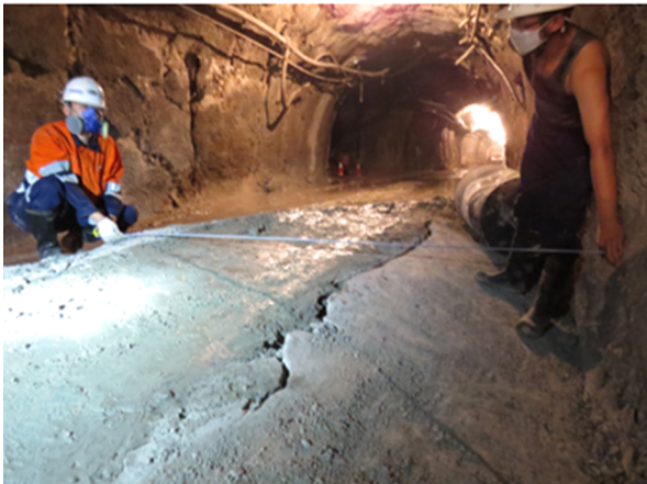
Fig. 10 Floor heaves of roadways by different supporting system: a roadway supported by steel arch, sprayed concrete and short bolts; b roadway supported combined supporting system
