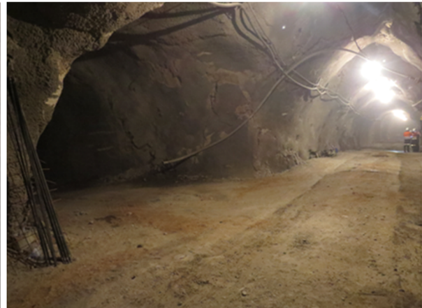
Fig. 10 Floor heaves of roadways by different supporting system: a roadway supported by steel arch, sprayed concrete and short bolts; b roadway supported combined supporting system
