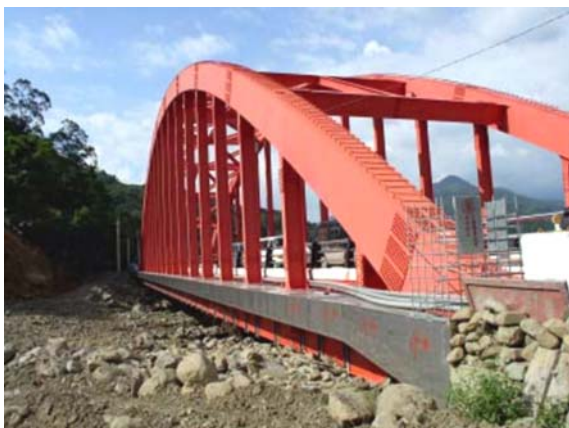
Fig. 17 Debris-flow deposit up to bottom of new arch-bridge
