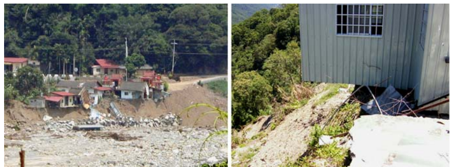
Fig. 10 Erosion increased the slope angle to critical conditions
