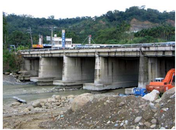
Fig. 22 Approximately 1 meter of bedrock (shale) removed beneath foundation
