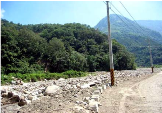
Fig. 20 River channel filled with debris overflowed into adjacent roadway
