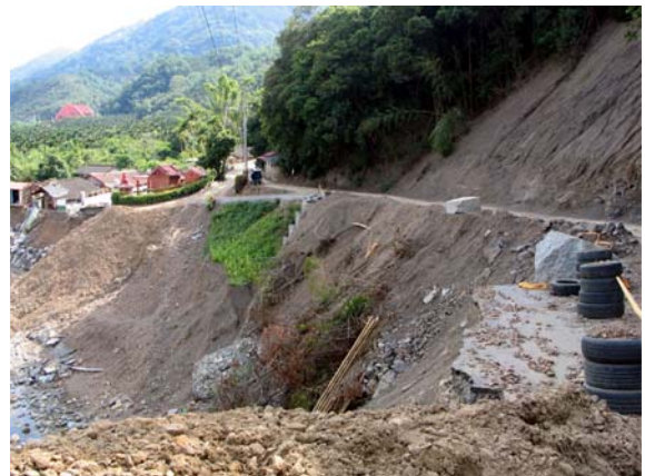
Fig. 18 Road damaged by slope failure
