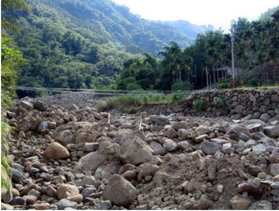
Fig. 19 Debris piled up and blocked waterway
