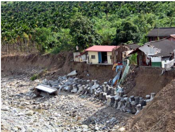
Fig. 10 Erosion increased the slope angle to critical conditions
