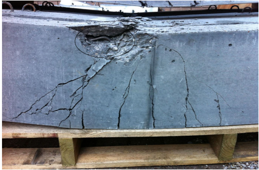
Fig. 14 C85 + 0.2 % SF beam B2 (Fig. 11) at failure when the mid-span deflection to span ratio had reached 60/1500. Note the buckle in the longitudinal compressive reinforcing bar which was accompanied by a drop in the load (Fig. 11). This was an exception observed only in one beam out of the nine tested
