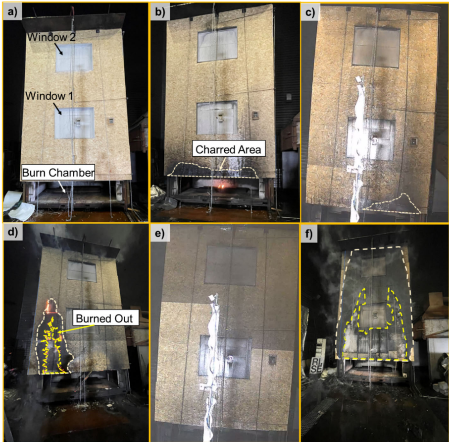
Figure 6. Post-fire damage on the façade. (a) Pre-fire condition. (b) 3 WM. (c) 3 WM with plates. (d) 1 WM with plate. (e) Sprinkler. (f) Freeburn. Light yellow lines represent the borders of the charred areas, while yellow lines show the burned-out areas (Color figure online).
