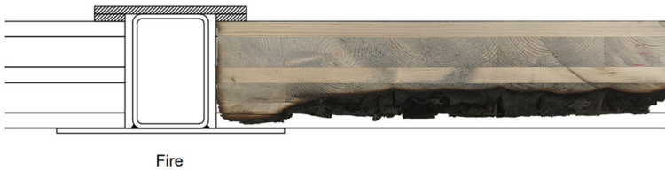
Figure 7. Charring of a CLT panel supported by a fire-protected steel beam at 61 min of fire exposure.
