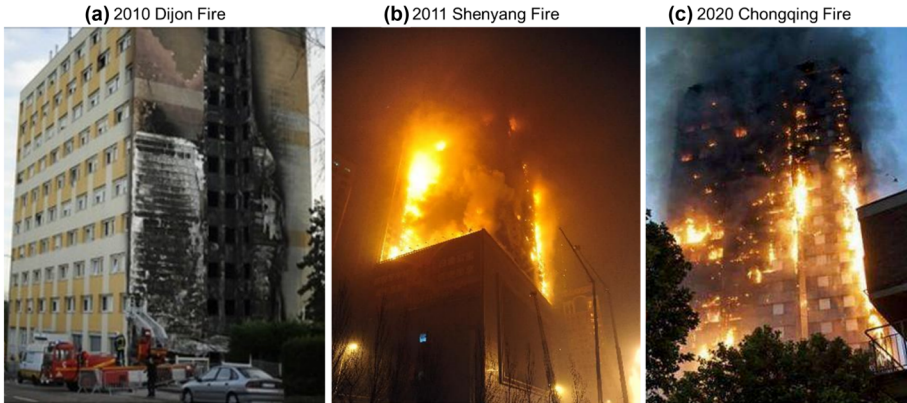
Figure 1. Typical EPS ETICS facade accidents, a Dijon fire, France in 2010 https://www.bbc.com/news/world-europe-11752303 , b Shenyang fire, China in 2011 http://news.sina.com.cn/c/2011-02-08/153321924087.shtml , and c Chongqing fire, China in 2020 http://cmszfb.oss-cn-beijing.aliyuncs.com/u/cms/www/202001/02143433gso9.jpg .
