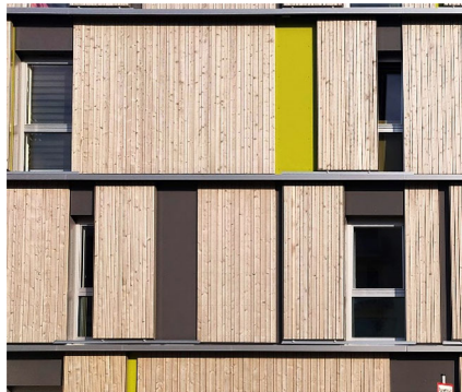
Figure 24. Façade as vertical tongue and groove cladding.
