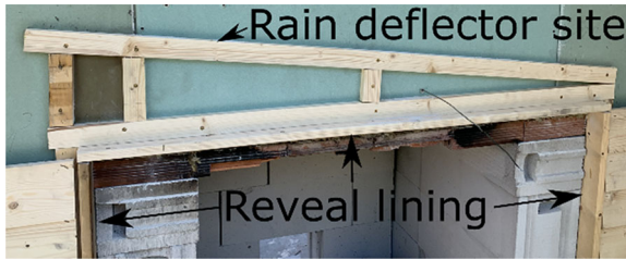
Figure 28. Reveal lining and rain deflector site.
