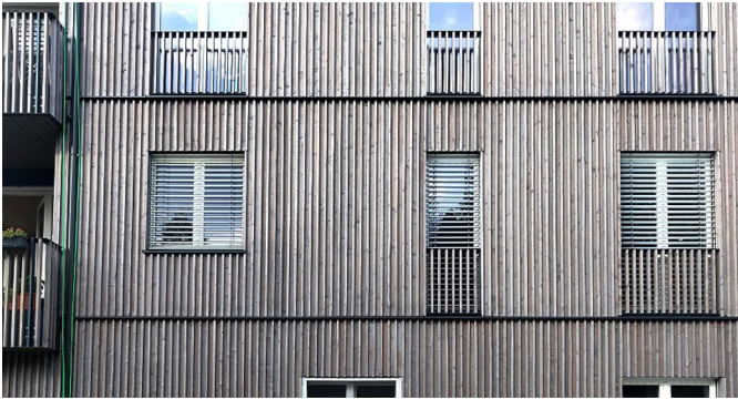
Figure 23. Façade as vertical cover strip cladding.
