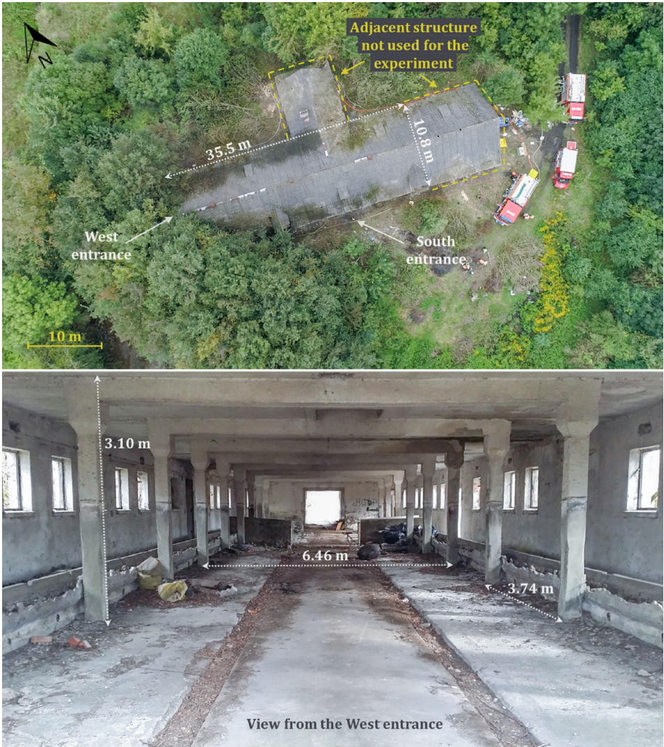
Figure 2. Plan view photograph of the building (top) and internal view of the compartment (bottom) of 'Obora' where the x-ONE experiment was carried out taken before the set-up of the experiment.
