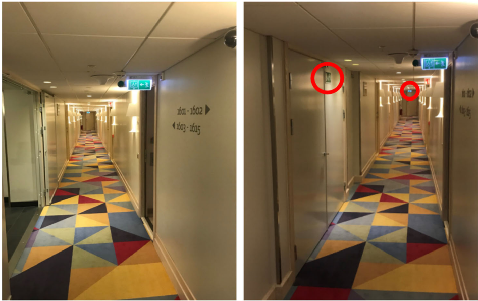
Figure 2. The hotel corridor with the double doors to the elevator lobby open (left) and closed (right). In the right image, the fluorescent evacuation sign on the elevator lobby door and the evacuation sign to the staircase at the end of the corridor has been circled.
