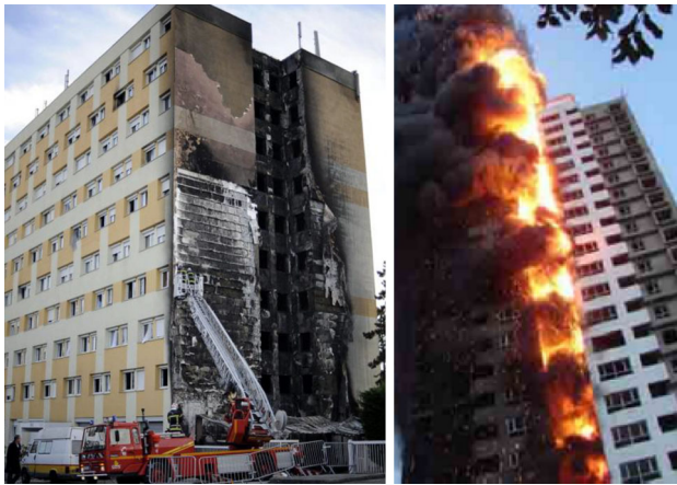
Figure 1. Real fire propagation of vertical U-shape building façade in France (left) and in China (right) both occurred in 2010.
