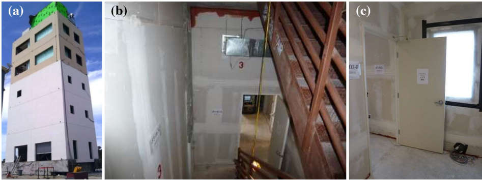
Figure 3. Photographs of (a) the façade systems on the BNCS test specimen, (b) stair enclosure looking onto Floor 3, and (c) partition wall and door on Floor 3 [19, 23].
