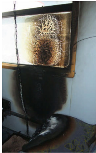
(c) view of the window and wall panel
