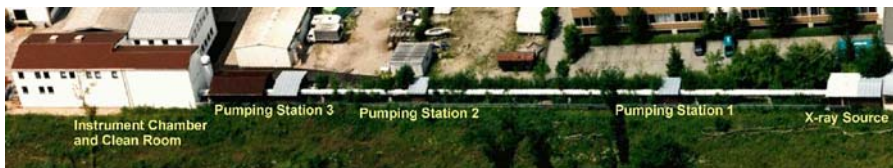
Fig. 2 Overview of the X-ray Test Facility PANTER situated in Neuried in the southwest of Munich, with a 123 m vacuum tube connecting the X-ray sources (located to the right) and the instrument chamber (on the left of the image)
