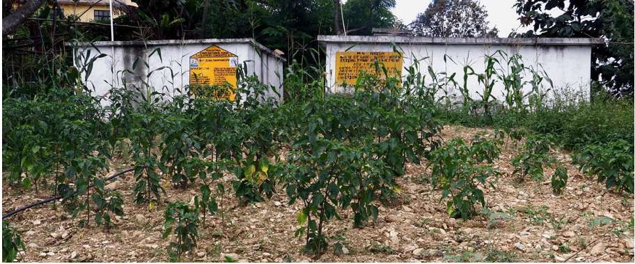
Fig. 2 Household livelihood assets (HLAs) like this 10,000-L reinforced concrete water storage tank built with an investment of about USD 1400 has enabled homestead farming
