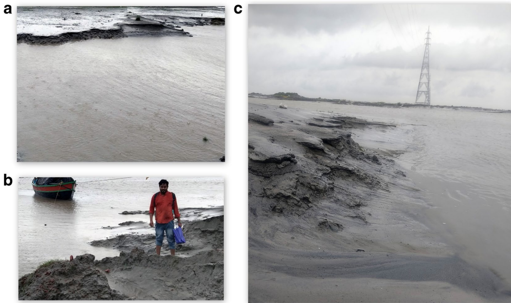
Fig. 22 Erosion at the Kakdwip sector near Kalinagar
