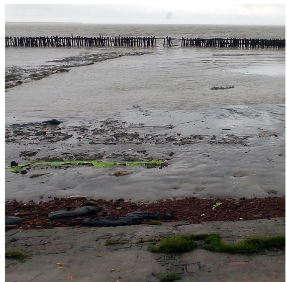
Fig. 24 Wooden embankment and brick kiln at the Kakdwip sector
