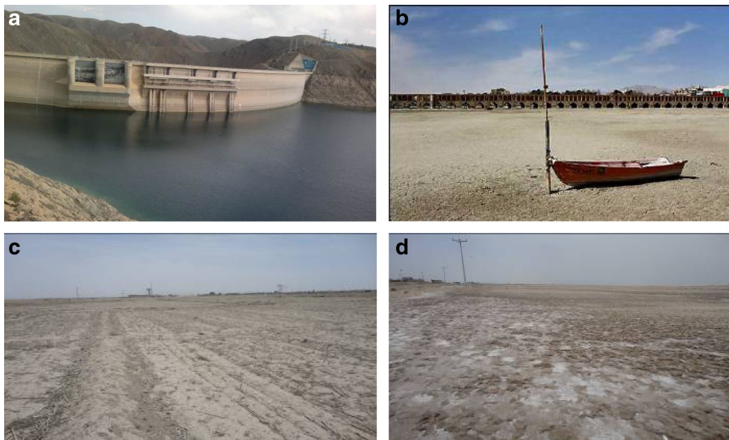
Fig. 3 Zayandehrood Dam and its effect on desertification. Photographs of a Zayandehrood dam, b Zayandehrood River, c abandoned agricultural land, and d salinized agricultural land
