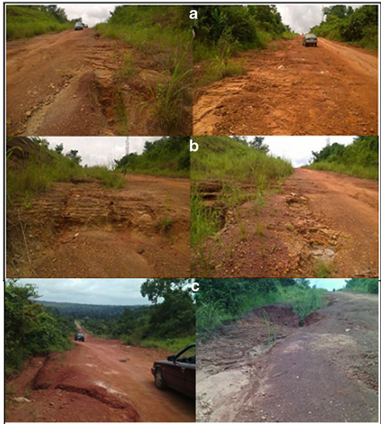
clearing out, and weak road bed stabilization could cause erosion and water logging along the highway alignment and surrounding bushes (Fig. 11) and thereby triggering creeping of the clays through clay mineral activity and increased pore pressures within clay layers. The provision of surface drainage systems and the completion of the other mentioned construction services would go a long way in the maintenance of the highway and thus increase
