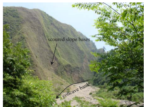
Fig. 11 Scoured slope bases next to the concave banks of river
