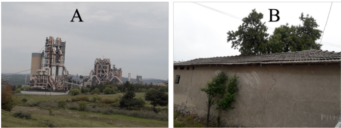
Fig. 1 a Cement plant in Ezine-Canakkale. b Cement dust accumulated on the roofs of the houses
