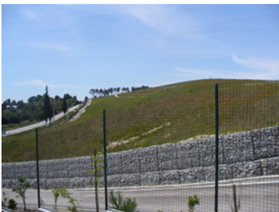
Fig. 8 Urgeiriça mine the pile of wastes in the Barragem Velha, after rehabilitation works
