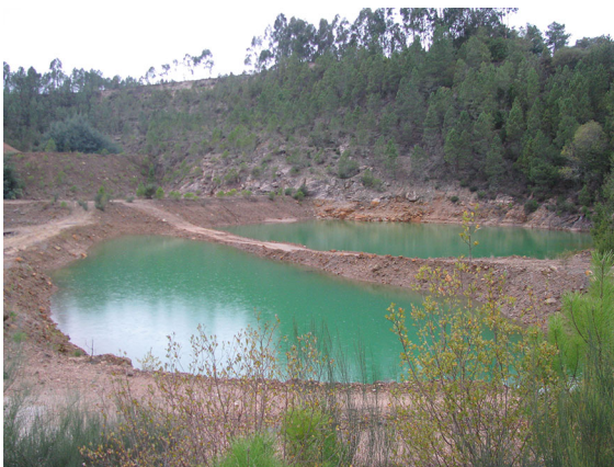
Fig. 6 Quinta do Bispo uranium mine: aspect of the open pit filled with effluent
