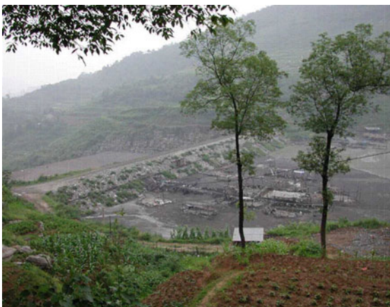
Fig. 3 View of ore-tailing reservoir
