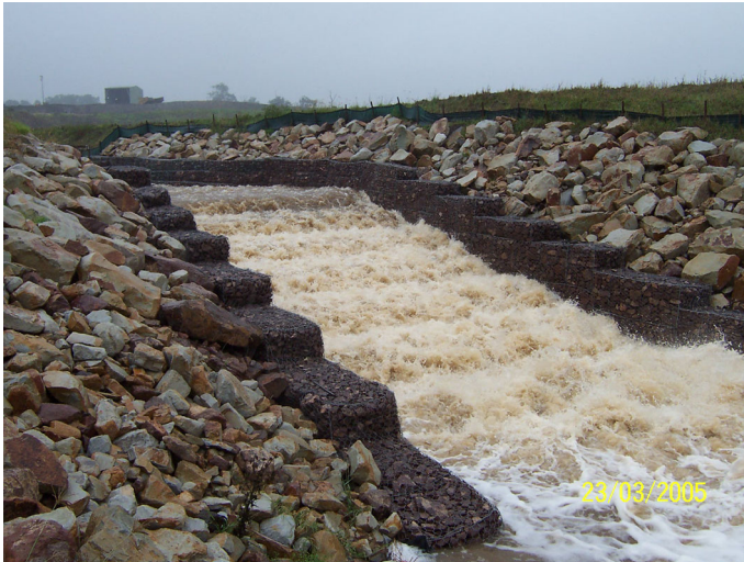
Fig. 1 Aeration above a gabion stepped chute at Duralie Coal project (Australia) on 23 March 2005 (Courtesy of Tony MARSZALEK)
