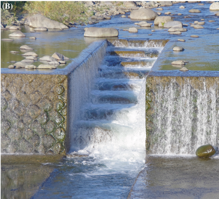
Fig. 1 Photographs of pooled stepped structures. a Pooled stepped spillway of Le Pont dam (France) in June 1998— Left looking downstream, Right looking upstream. b Fishway structure on the Okura River (Japan) on 9 October 2012—The stepped channel consists of a staggered combination of flat and pooled steps
