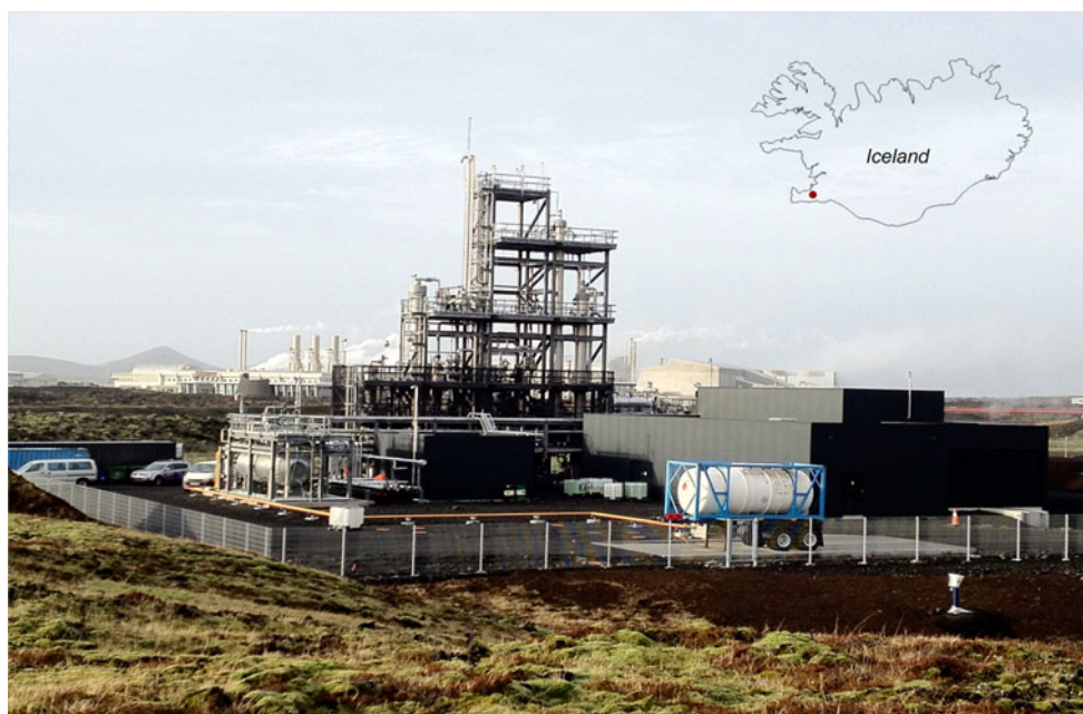
The “George Olah Carbon dioxide to Renewable Methanol Plant” of Carbon Recycling International in Iceland based on local geothermal energy. The first commercial carbon dioxide recycling plant operating in the world. “Reprinted with kind permission of K. C. Tran, CEO, Carbon Recycling International, Iceland”
