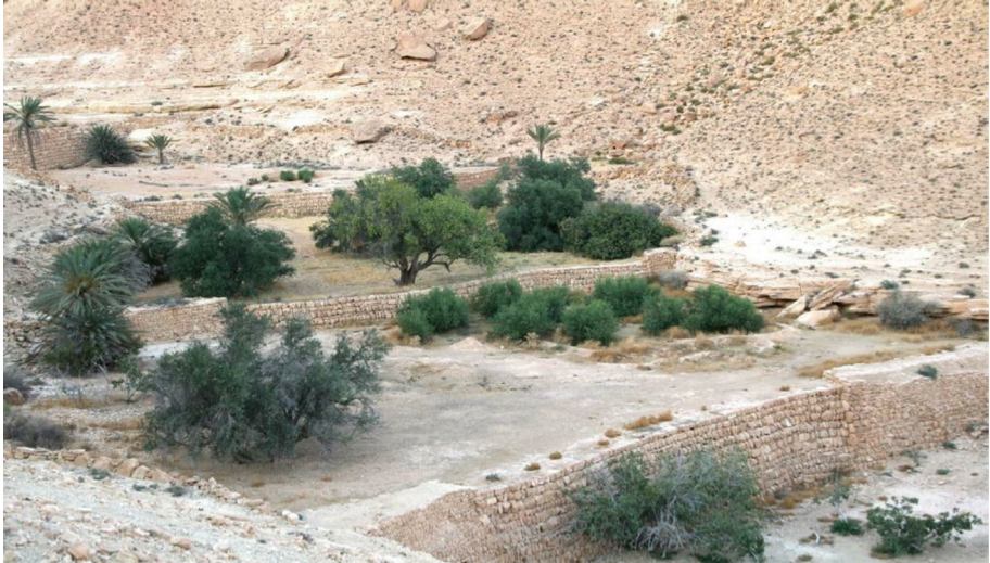
Fig. 6 Example of vegetation watercourse jessour. From the picture it is clear the drystone walls distribution along the water course and the way they are built. Most of the tree trunks are buried under layers of soil which have settled over the years
