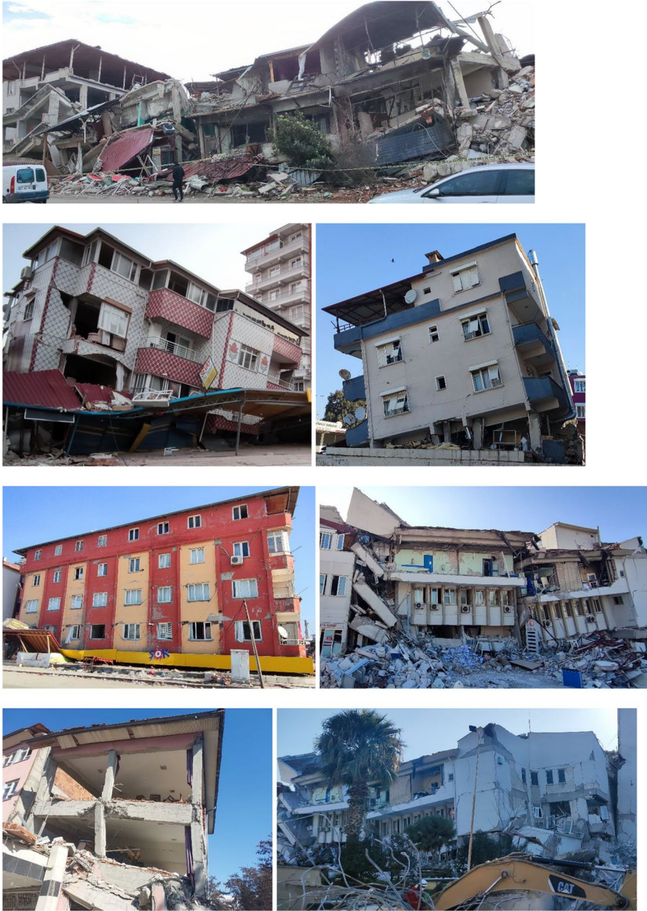
Fig. 7 Tilted or partially collapsed buildings
