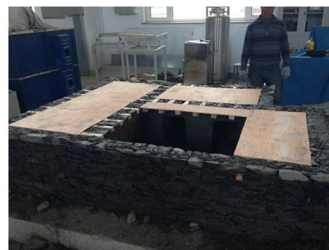
b. Beams and floor slab
