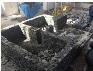
a. Masonry walls in the bottom base
