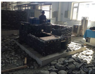
c. Masonry walls on the second floor
