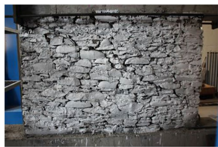
(b) The joints of the wall gradually loosened
