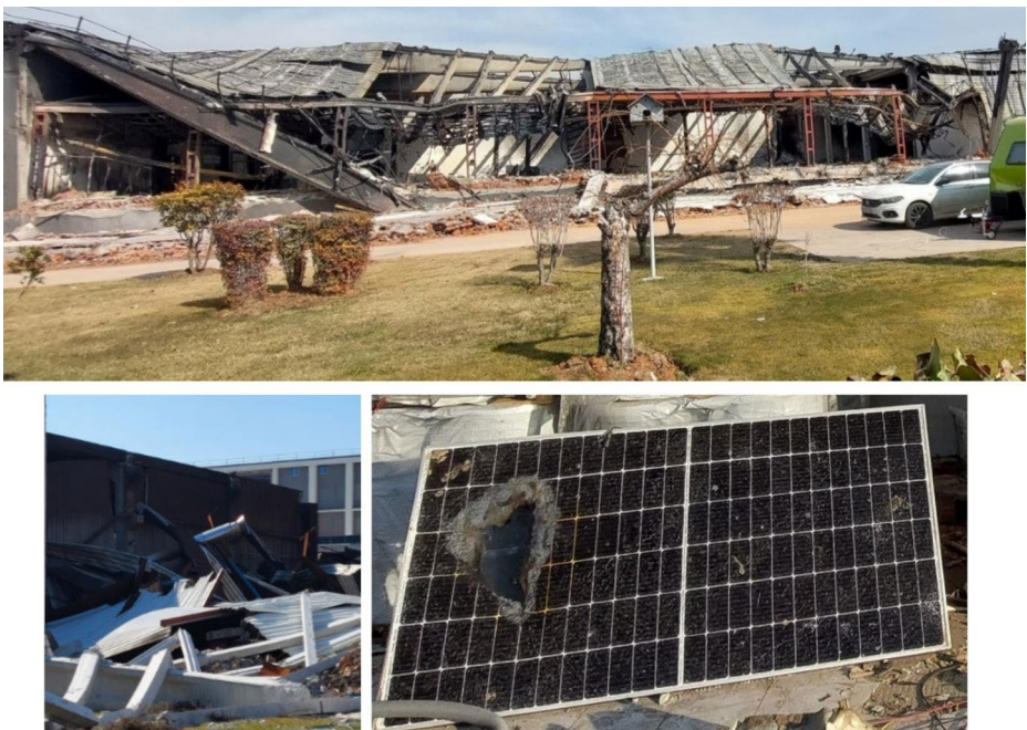
Fig. 17 Incidents of fires following earthquakes observed in Dulkadiroglu (top) and Turkoglu (bottom)
