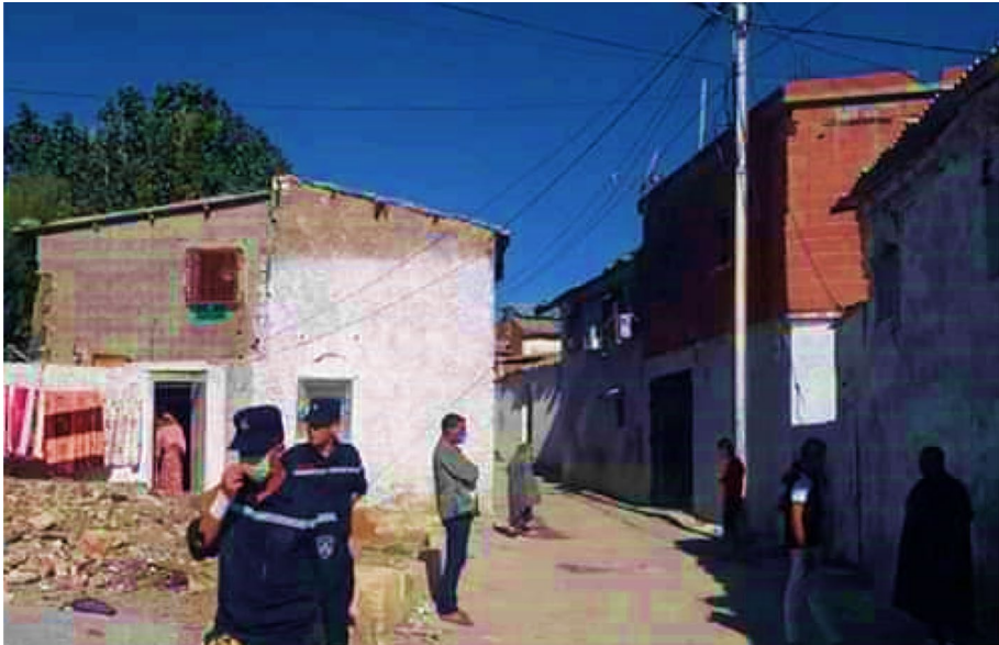
Fig. 8 Insertion of new concrete constructions "within" existing blocks during the building process and at the end
