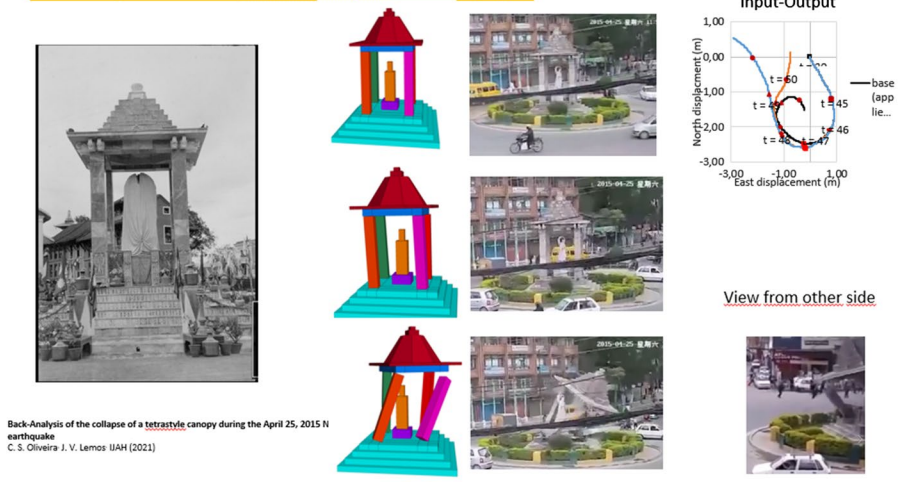
Fig. 83 Back-analysis of a collapsed tetrastyle canopy
