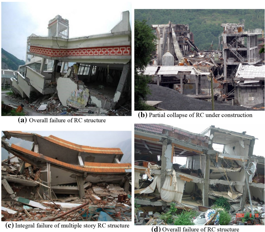
Fig. 5 Failure of RC structure
