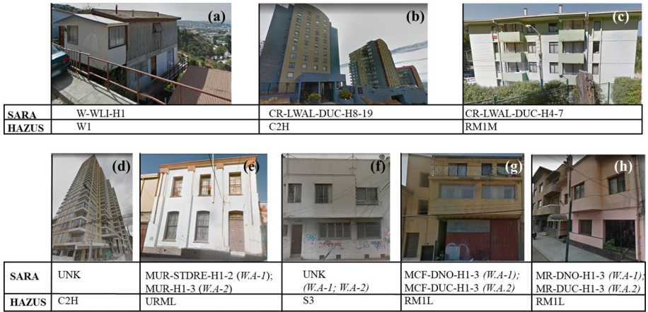
Fig. 3 Pictures of some selected buildings’ façades surveyed in Valparaíso. Their classifications in terms of the SARA and HAZUS schemes are displayed considering the two weighting arrangements presented in Table 3. No distinction is made when both weights led to the same class. ©Google Street View, digital images, 2021
