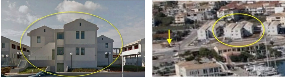
Fig. 1 The Lefkada Regional Administration building (yellow ellipse) and location of the free-field accelerometer (yellow arrow)
