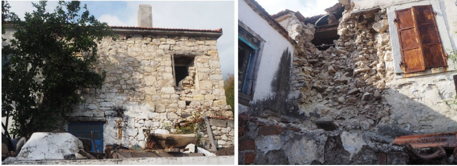
Fig. 16 Typical masonry wall in Kösedere and example of a collapsed wall
