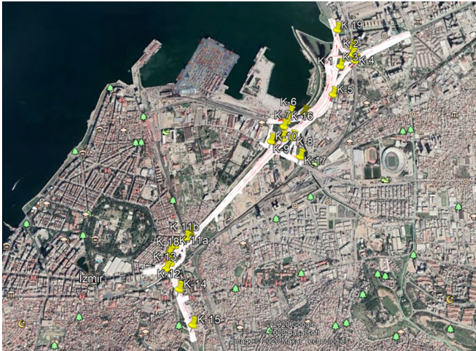
Fig. 18 The highway line selected and bridges assessed
