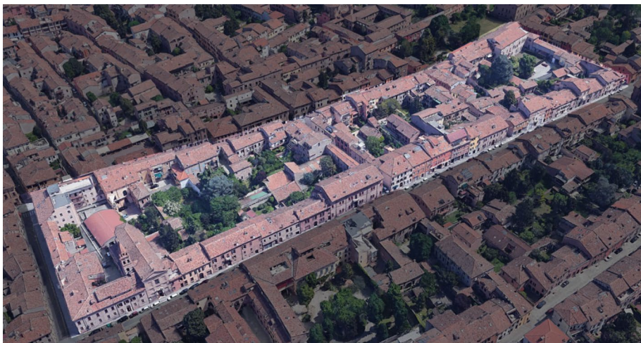
Fig. 1 The historical aggregate in the center of Ferrara, Italy (aerial view)
