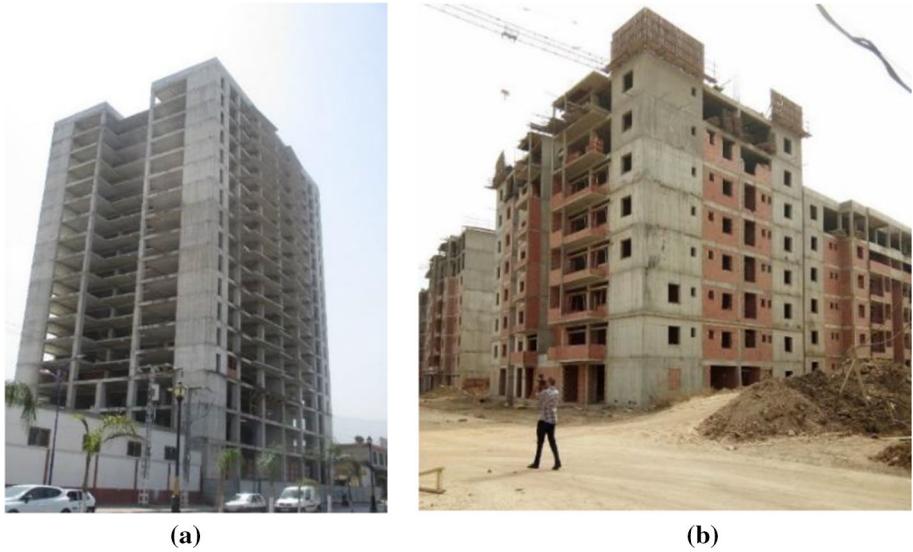
Fig. 2 Typical high-rise dual RC system MRF-SW buildings in Blida
